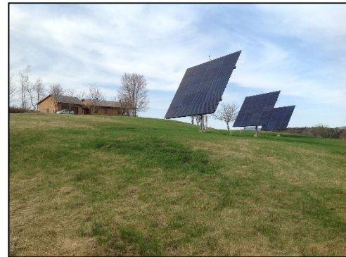
Figure 1: Small scale solar -- 15 kW
